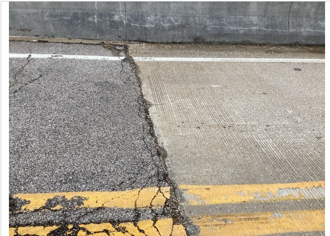
Span 1 spall
