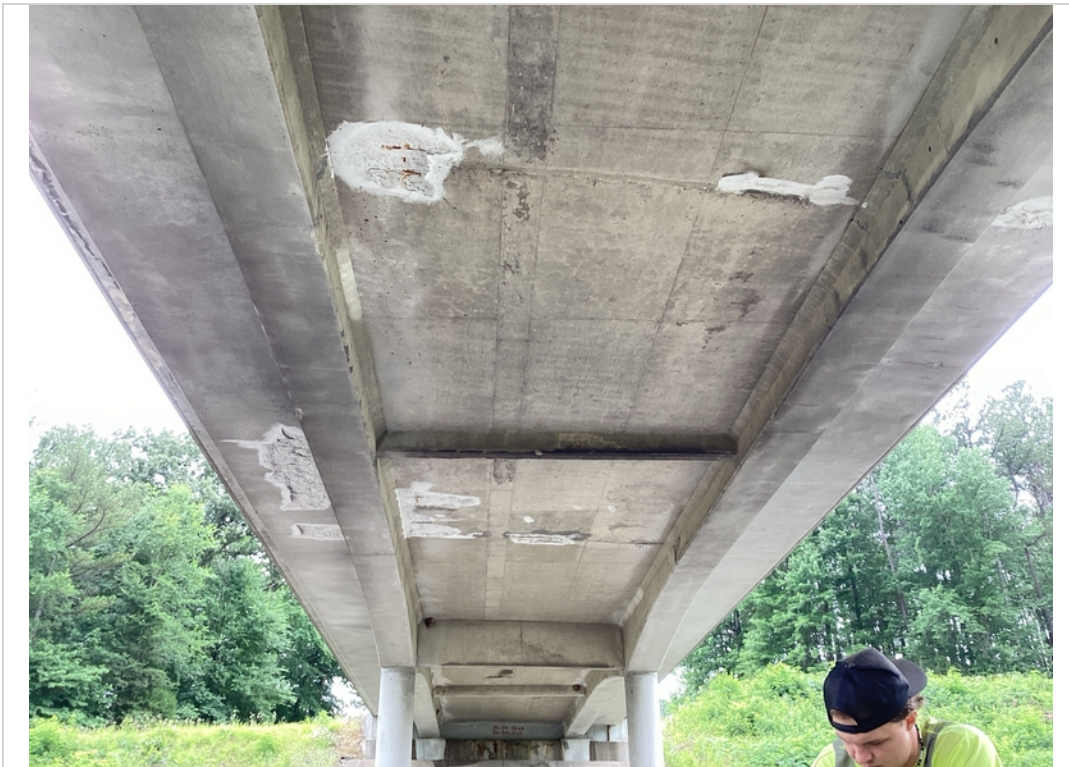
Bottom deck of span #2
