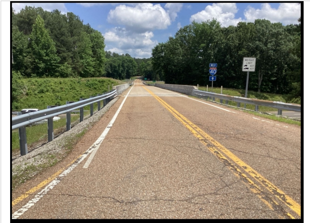
Approach 1 weight limit sign @ 26.47 bridge
