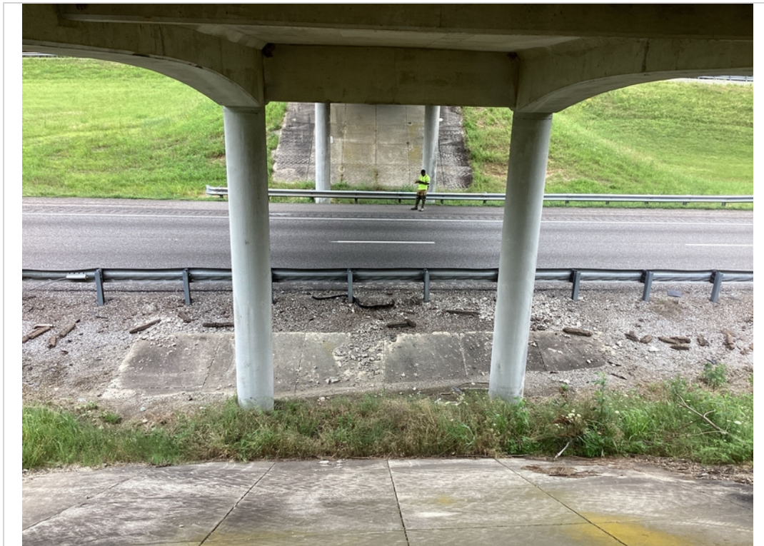
Bent #1 looking forward
