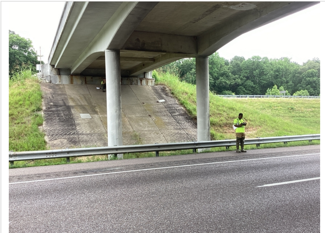
Bent #2 looking forward
