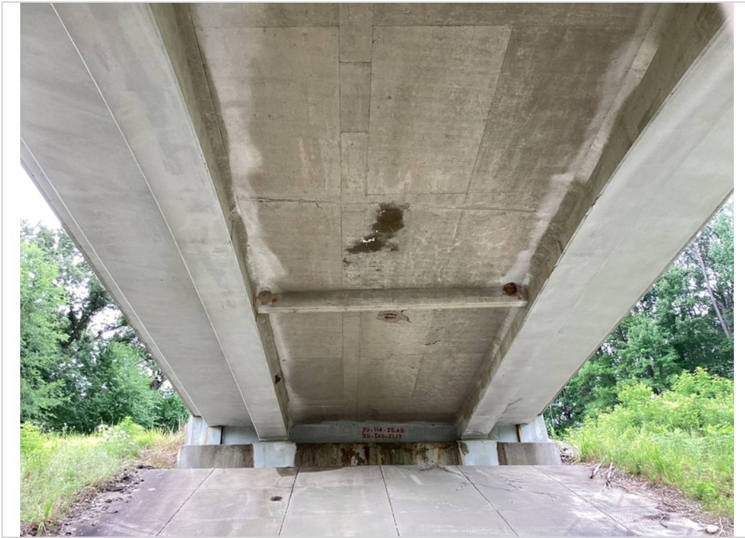
Span 1 bottom deck typical
